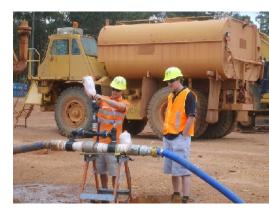
Powder is mixed into a water cart at a predetermined concentration using a Eductor. This is done as the water cart is being filled and once set up should not impede on the length of time taken to fill the water cart. Once the powder has been mixed into the water to form a co-polymer then the product is used as if it were normal water and no deviation from common practice is required, basic Rip and Re-compact methodology applies.
